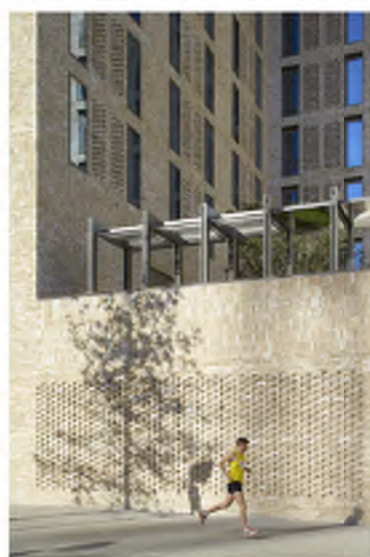
Light brown brick facade
