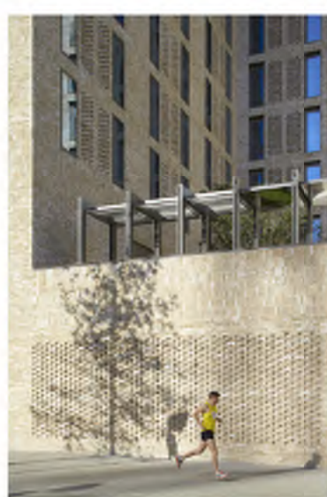
Light brown brick facade
