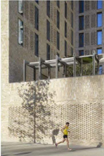
Light brown brick facade
