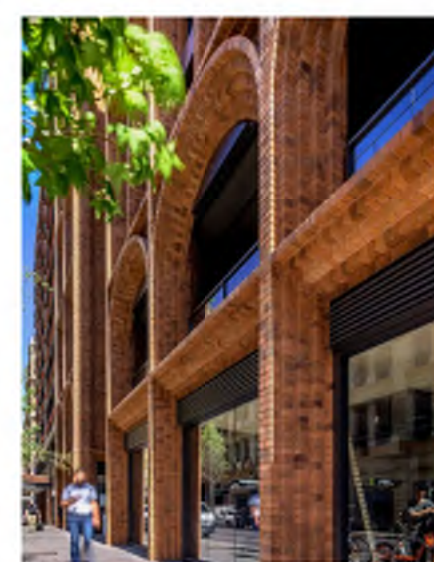
Dark brown brick facade
