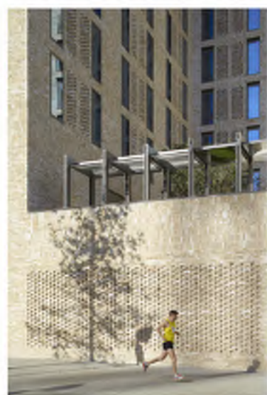
Light brown brick facade
