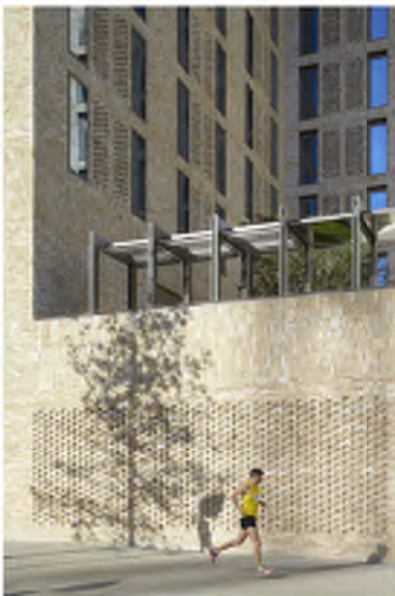
Light brown brick facade
